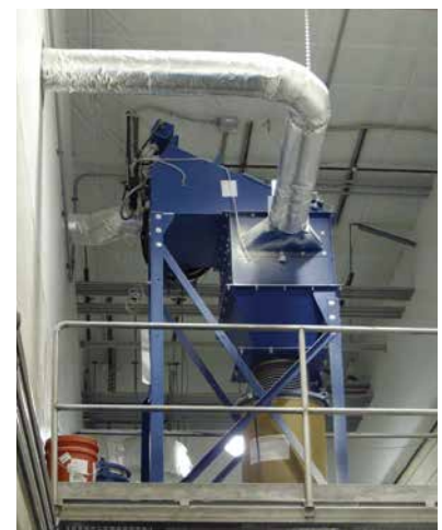
CPC-3 - Powdered milk dust in cheese factory 1,200 cfm (2,038 m 3 /h)
