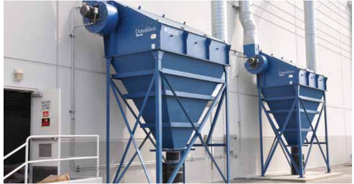
CPC-24 - Paper tissue manufacturing 7,600 cfm (12,910 m 3 /h)
