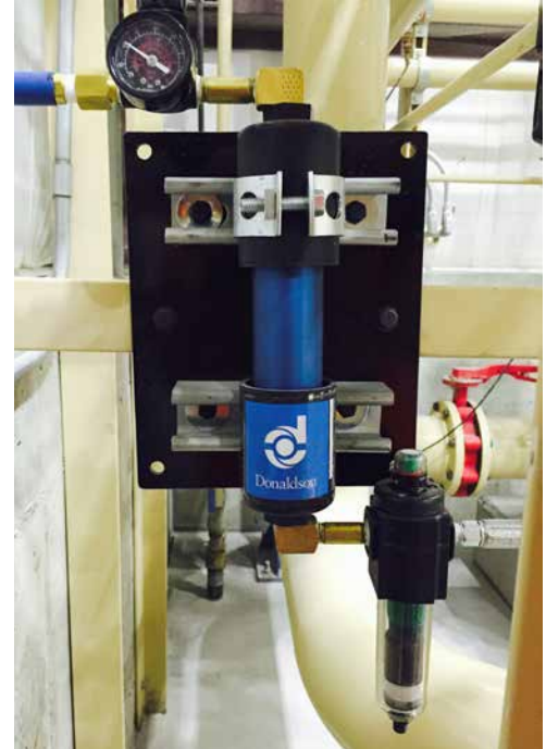
The Reservoir Air Dryer is not recommended for use on gasoline holding tanks or for the head space of any flammable liquid (Flash Point of 38°C / 100°F)
